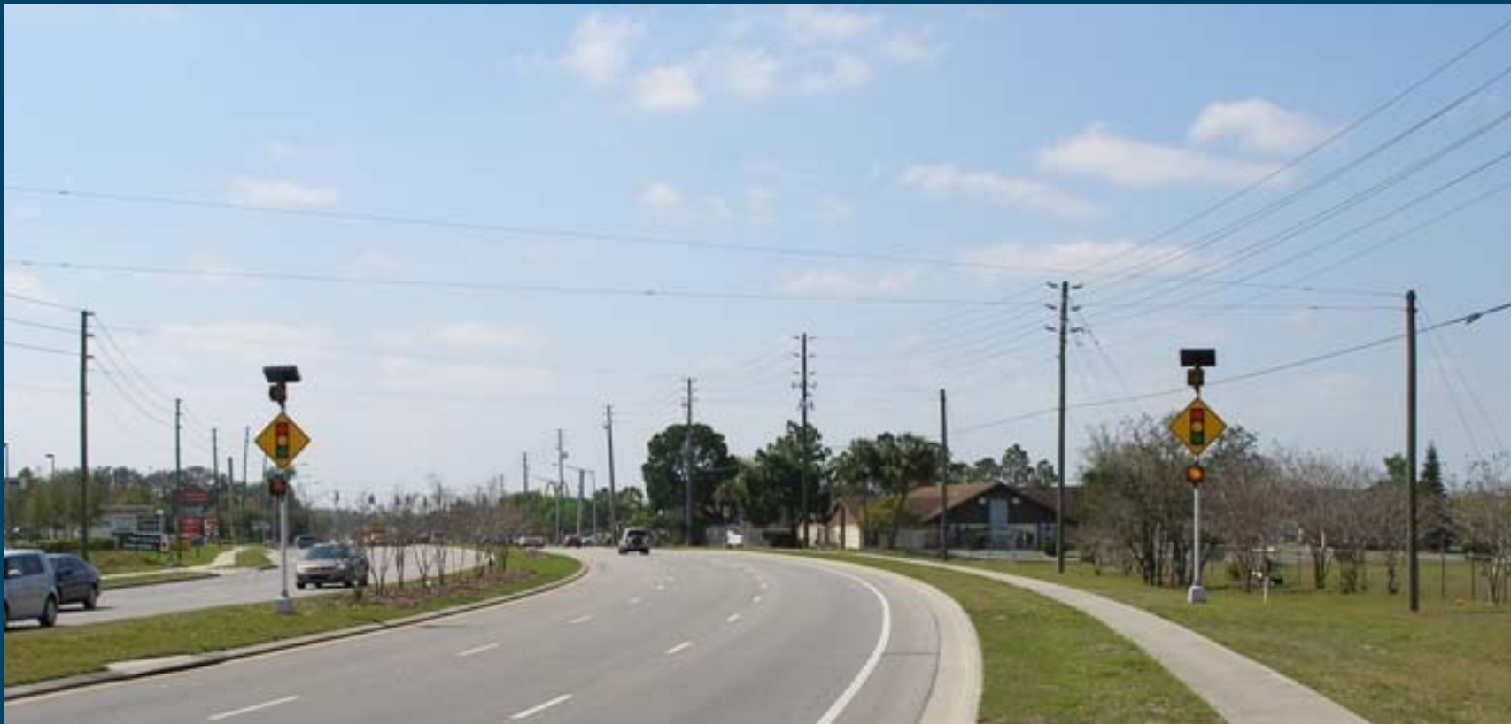
Signal Ahead signs with solar-powered flashers
